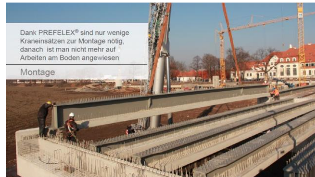
Figure 18: Installation [C+P Brückenbau GmbH & C. KG, Bad Homburg]
