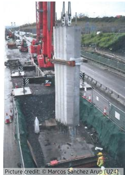
Figure 20: Connection of prefab pier elements to footing in a M50 extension bridge in Ireland
