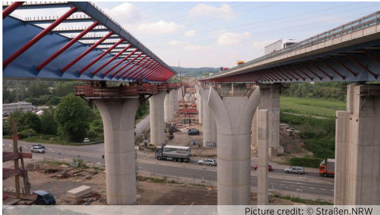
Figure 22: prefabricated covering pier parts for Lennetal bridge near Hagen
