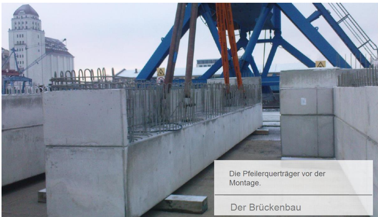
Figure 19: cross girder before installation [C+P Brückenbau GmbH & C. KG, Bad Homburg]
