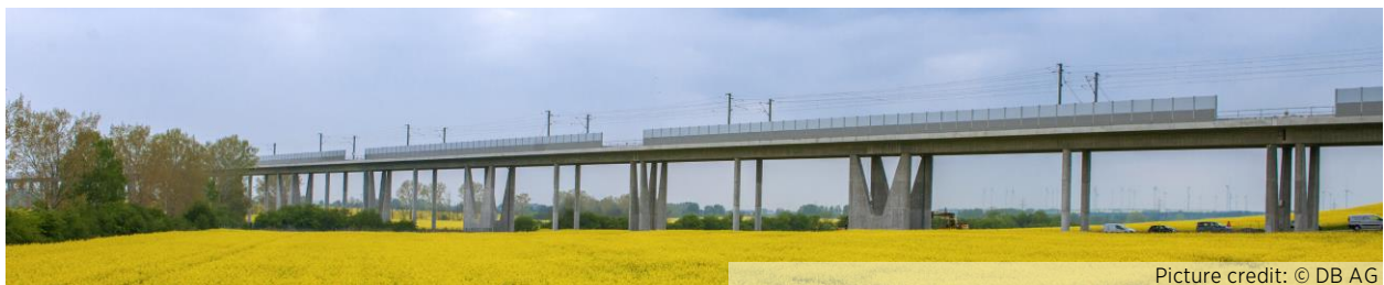
Figure 3: Gänsebach valley Viaduct during installation of noise protection
