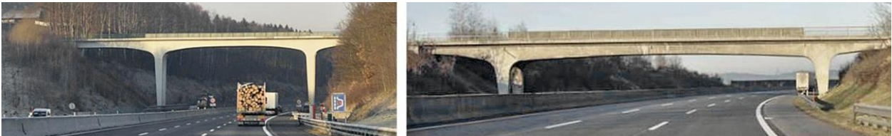
Figure 9: Different perceptions of two similarly dimensioned frame beams [U25]
