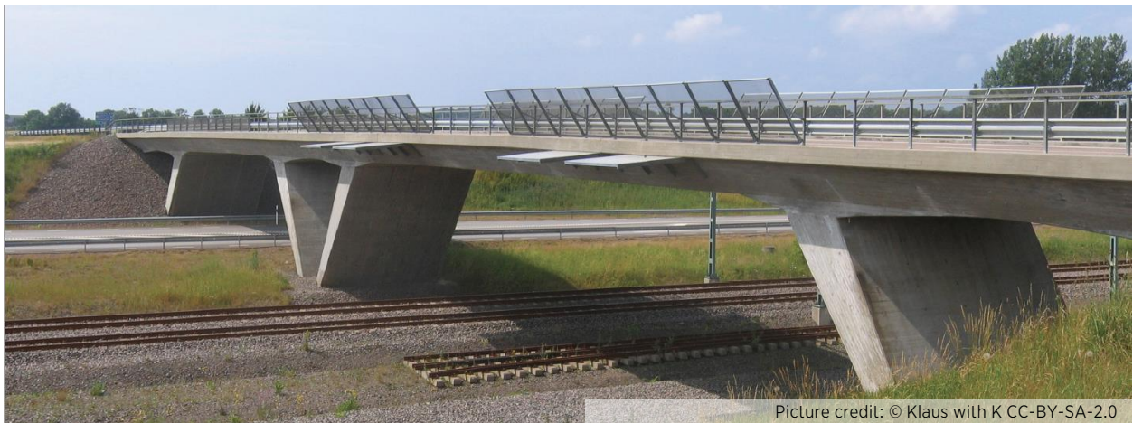
Figure 32: overhead catenary protection system to protect Railway and pedestrians
