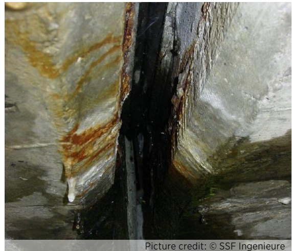
Figure 2: leaking expansion joint
