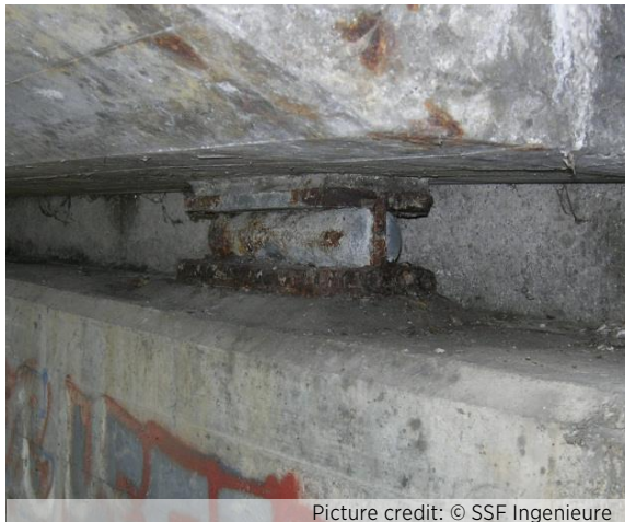
Figure 1: damaged bearing
