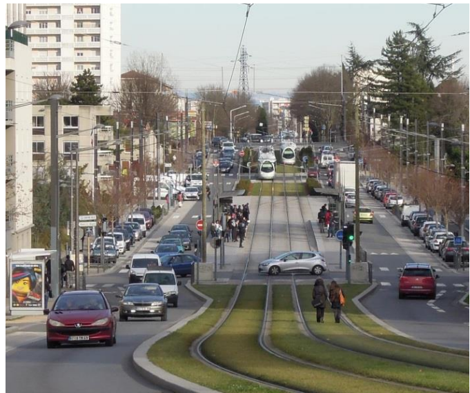
Figure 3.28: example of axial track position
