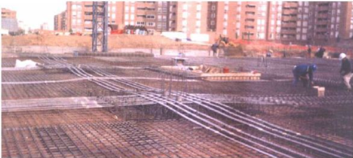
Figure 14.49: Post – tensioned concrete slab construction (Source: Internet)
