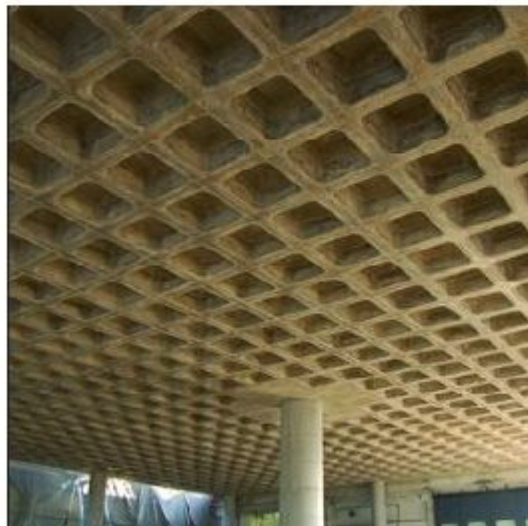
Figure 14.47 – waffle slab concrete (Source: Internet)
