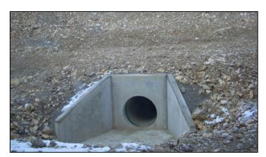
All the various headwalls shall include a cast in-situ cut-off wall, compulsorily poured in situ and in contact with natural ground. This shall be cast in-situ without formwork. This restriction applies also to prefabricated headwalls.
