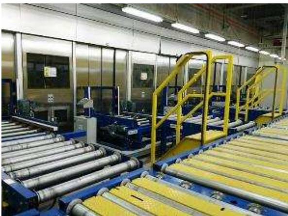
Luggage roller conveyor and luggage platform gate at the luggage platform on B3 level of A1 station.
