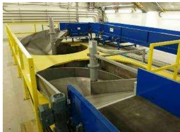
A conveyor belt and a spiral chute on B2 level of A1 Station.
