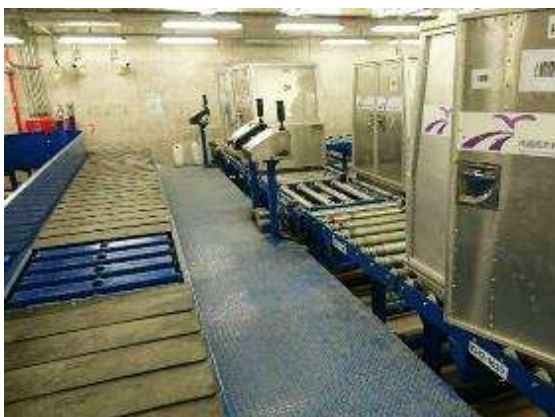
Luggage carousels, roller conveyors, and luggage lockers at the luggage area on B3 level of A1 station.
