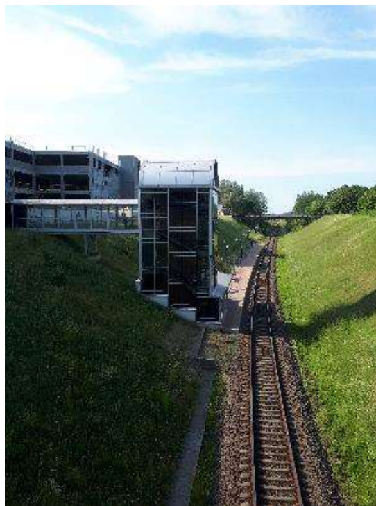
Illustration 44. Vilnius airport existing railway station (1520 mm track gauge)
