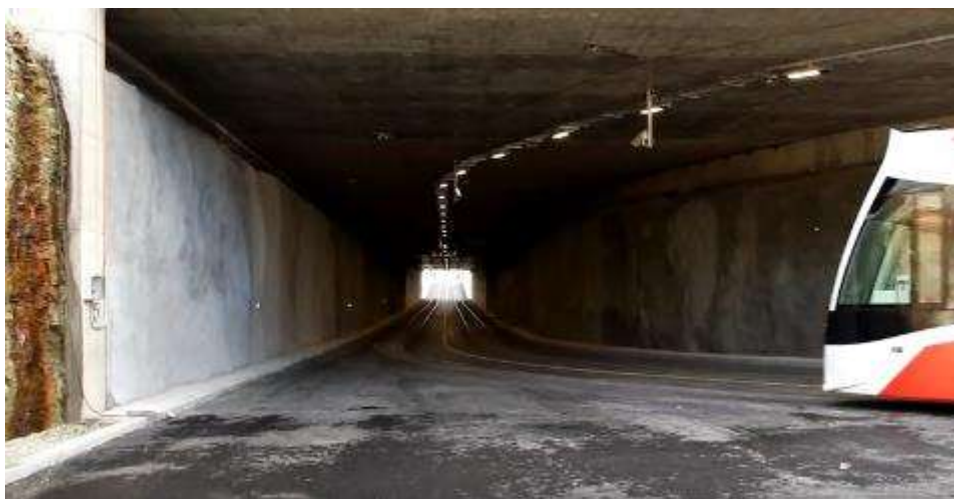
Illustration 38. Tramway underground passage
