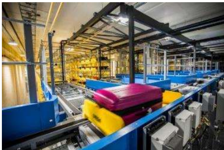
Illustration 1. Airport's luggage handling system (BHS)
